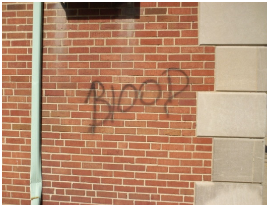
7357 Brookcrest – side of Roselawn Center Building
